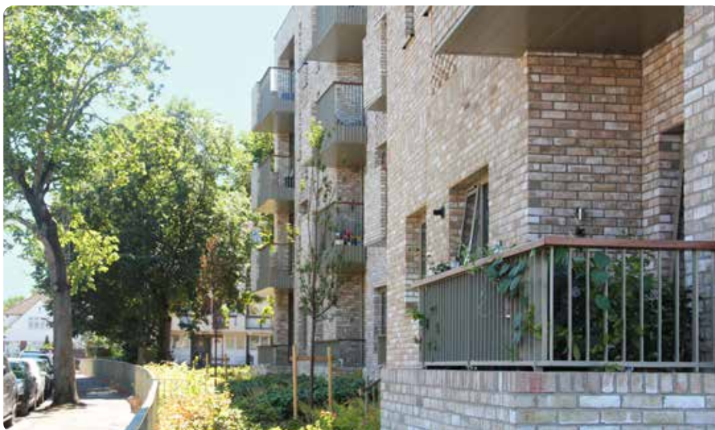
Extra care scheme with raised ground floor balconies set back behind planting
