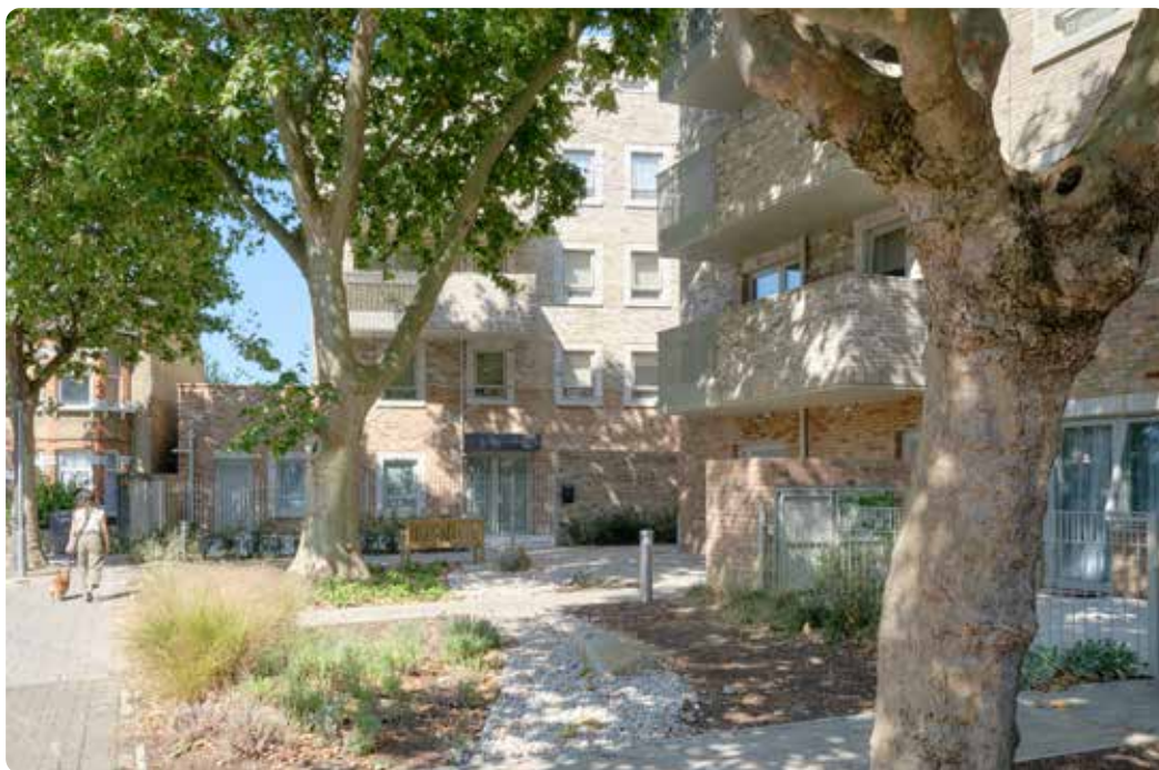
The simple form factor of this Passivhaus certified project is articulated with projecting balconies, brick garden storage and variations in brick colour
