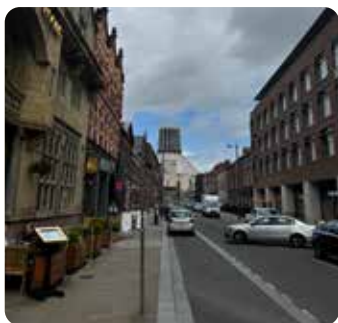
View of Liverpool Metropolitan Cathedral
