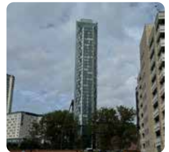
140m tall West Tower in the city centre
