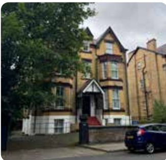
Four storey Victorian villas close to Sefton Park
