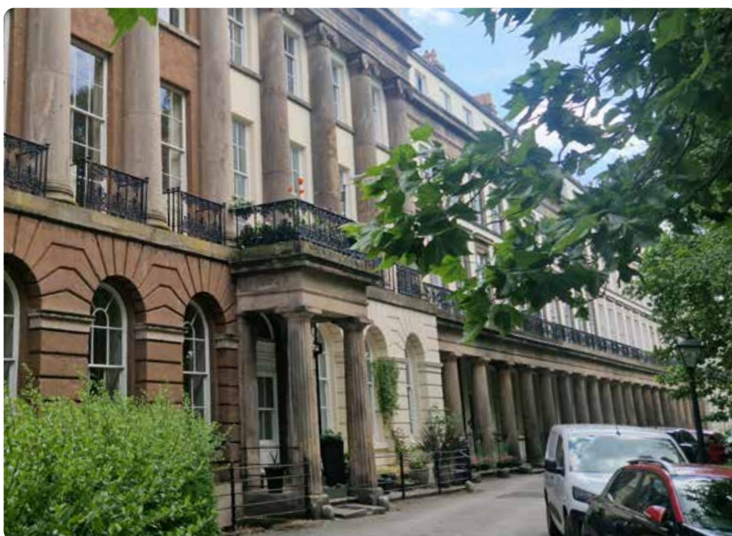
Retained, historic porticoes in Gambia Terrace
