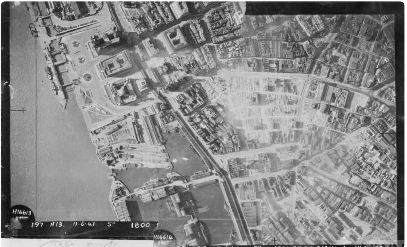
An aerial photo showing the extensive damage to the docks and commercial centre of Liverpool
