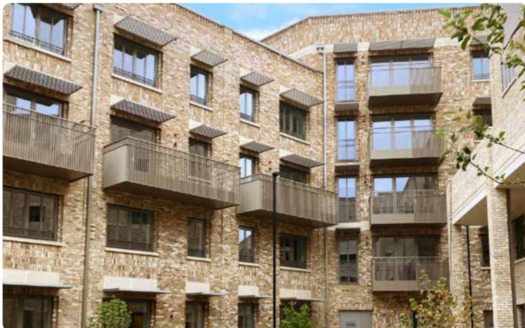
Balconies and fixed louvres on south facing windows provide shade for south facing windows
