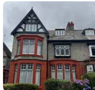
Three storey Victorian semi-detached with basement
