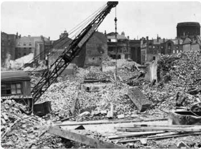
A photo of Lord Street, Merseyside after the fire damage from the May Blitz
